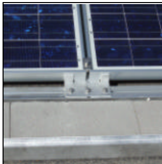
Bottom Bracket and Clamp
